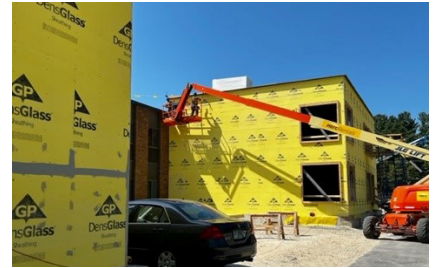
Above: Science Towers nearly closed in with exterior sheathing.
