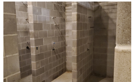
Above: Masonry being completed in locker room area.
